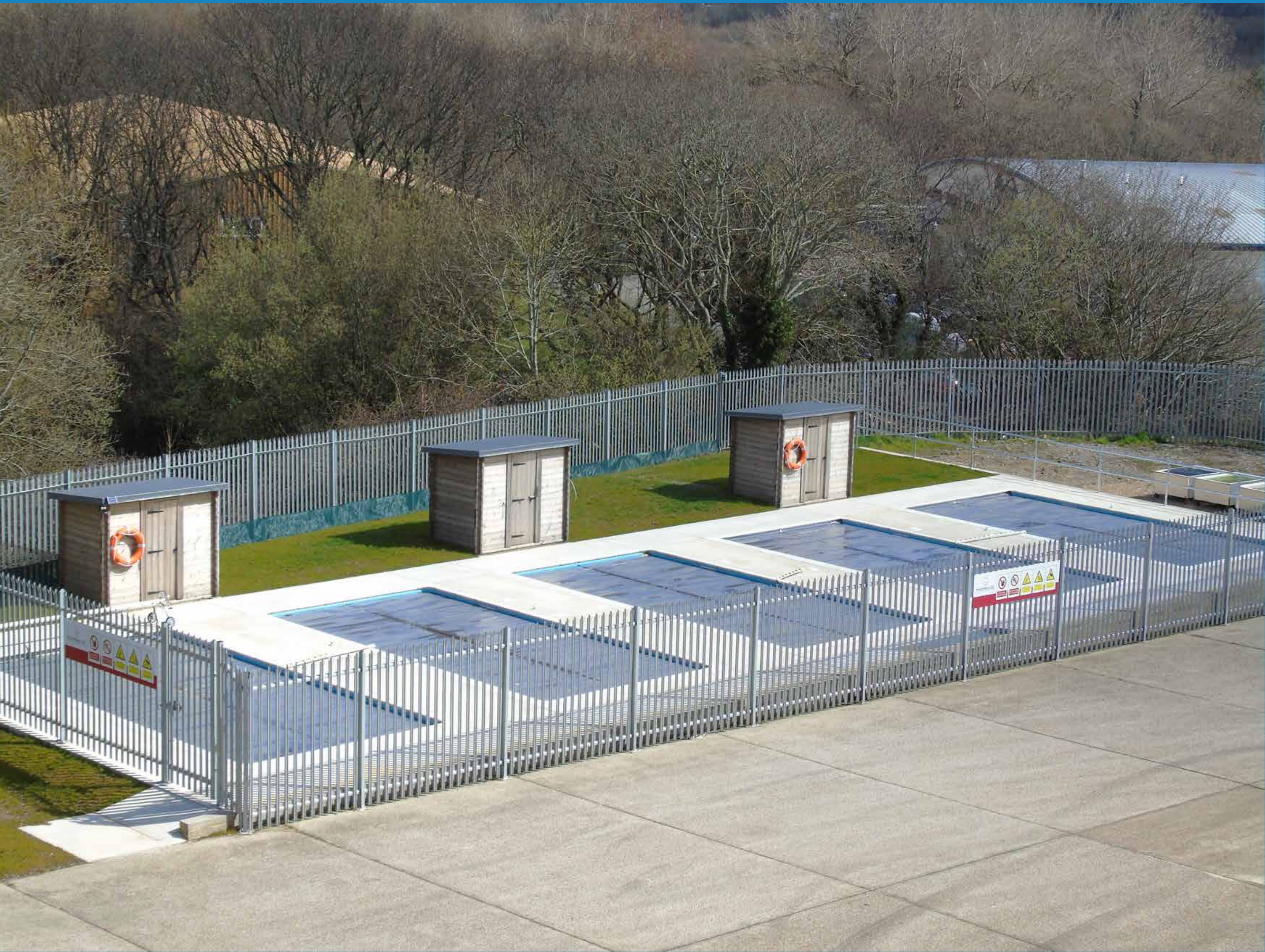
Figure 3. Bespoke testing facility, Plastipack Ltd, Hastings UK.
